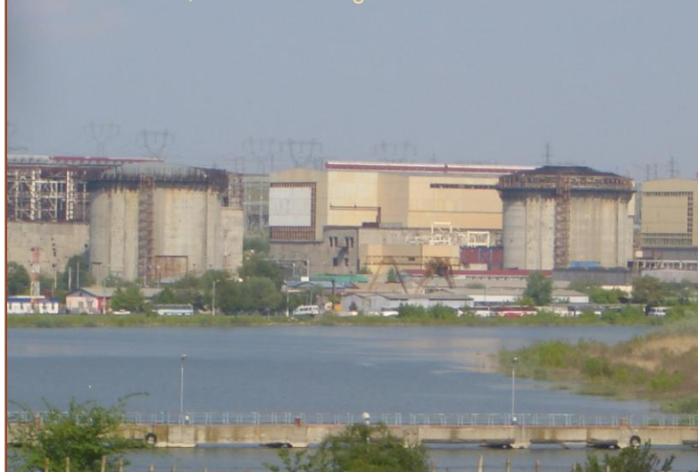
Cernavoda NPP, reactor buildings in conservation
