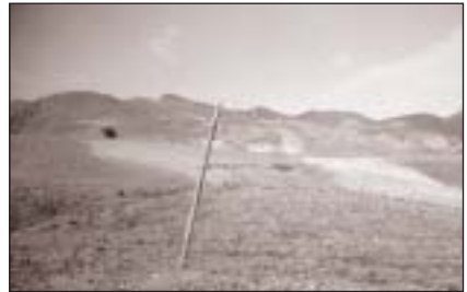
Scar left by the East Anatolian Natural Gas Pipeline (NGP) near Erzurum, north-eastern Turkey. The BTC pipeline would run alongside the NGP for 40% of its length in Turkey, between Erzurum and Sivas. (Greg Muttitt, PLATFORM)
