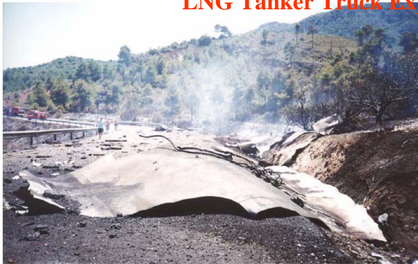
Fig. 4. Central part of the tank.
