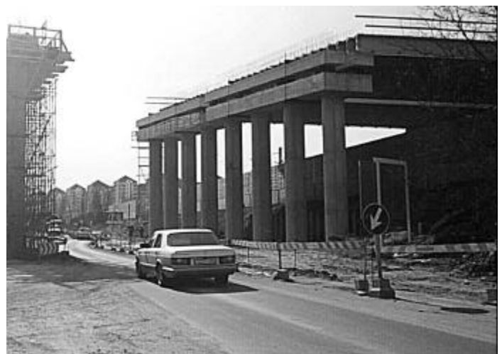
Construction of the motorway close to the houses
