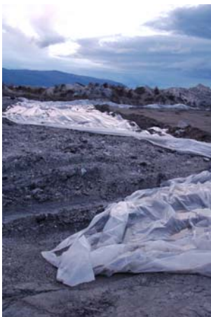
Soil encapsulation at the Coastal Terminal Site
