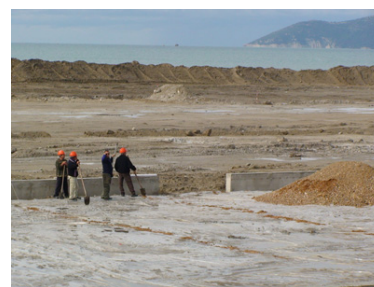
Construction works at the coastal terminal site
