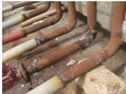
Image 2: Rusted pipes
