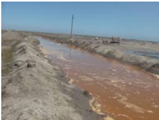
Image 3: The wastewater channel
