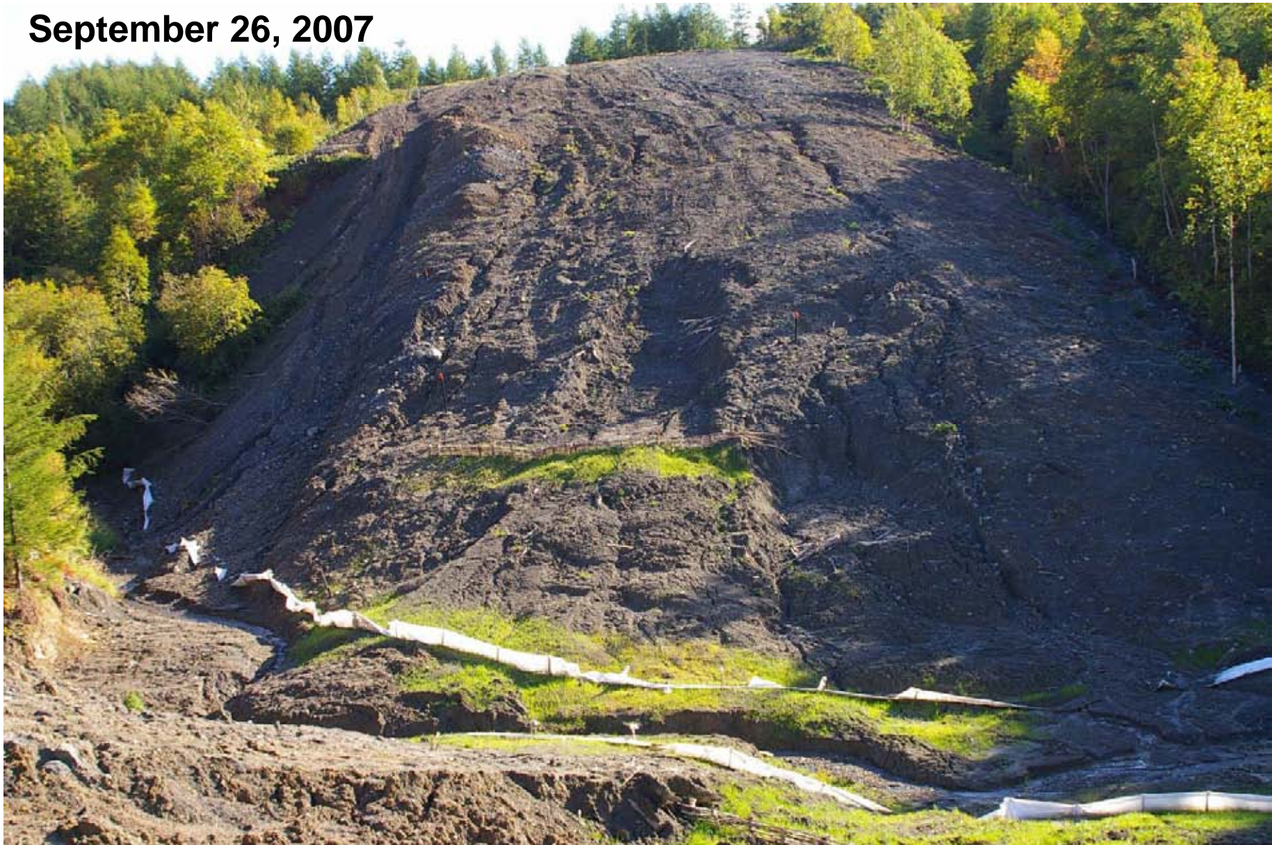
KP 461,0. The landslide on the left bank of the Krasnaya River right tributary. Dolinsk District. More than 4 months after the first land slide occurred on the slope, SEIC has not undertaken adequate, effective measures for control of land slides and erosion processes. Fences installed on the moving mud and very limited grass planting don't help at all.
