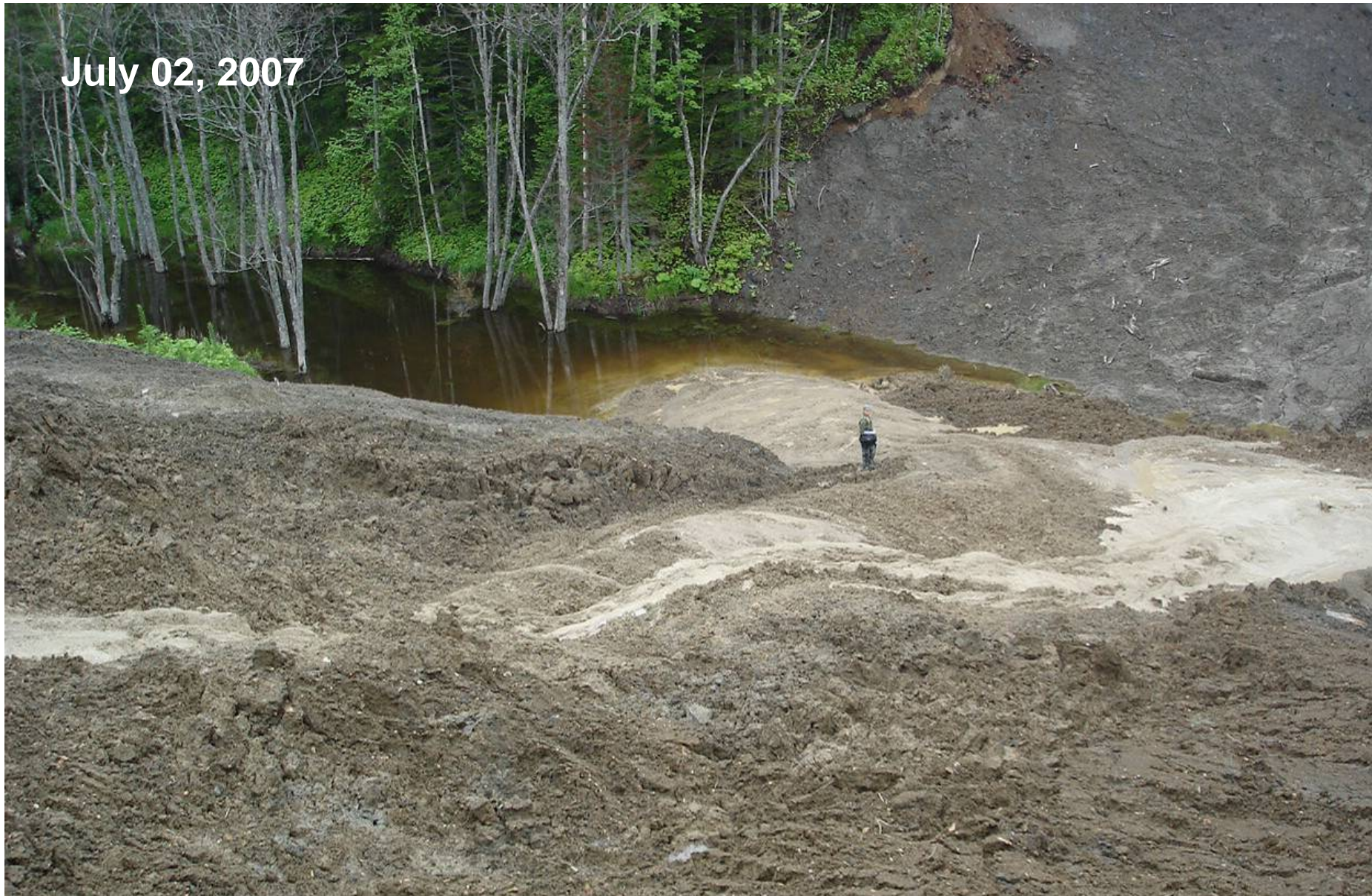
KP 462,6. The landslide on the right bank of the left tributary of the Baklanovka River, Dolinsk District. The landslide completely blocked the stream's bed, blocking water flow. An artificial pond has been created. Hydrological regime of the waterways was violated.
