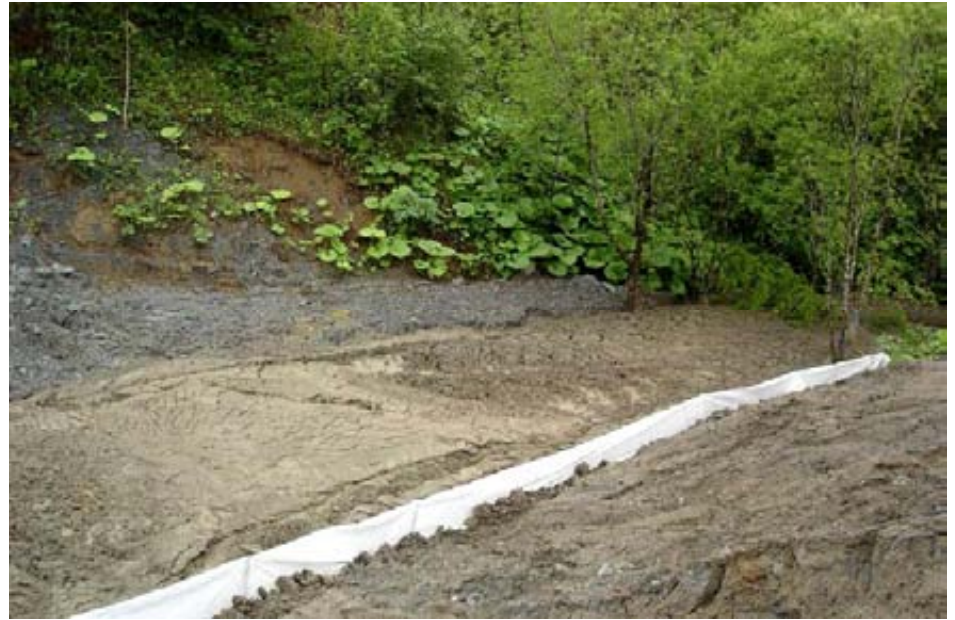
KP 461,0. The landslide on the right bank of Krasnaya River (the same place as on the previous slide). The photos above and below show that silt protection screens made of geotechnical fabric are mounted directly on the moving “bodies” of the landslides moving to the waterways. Photo above to the right - there is slush moving instead of the water. July 2, 2007.
