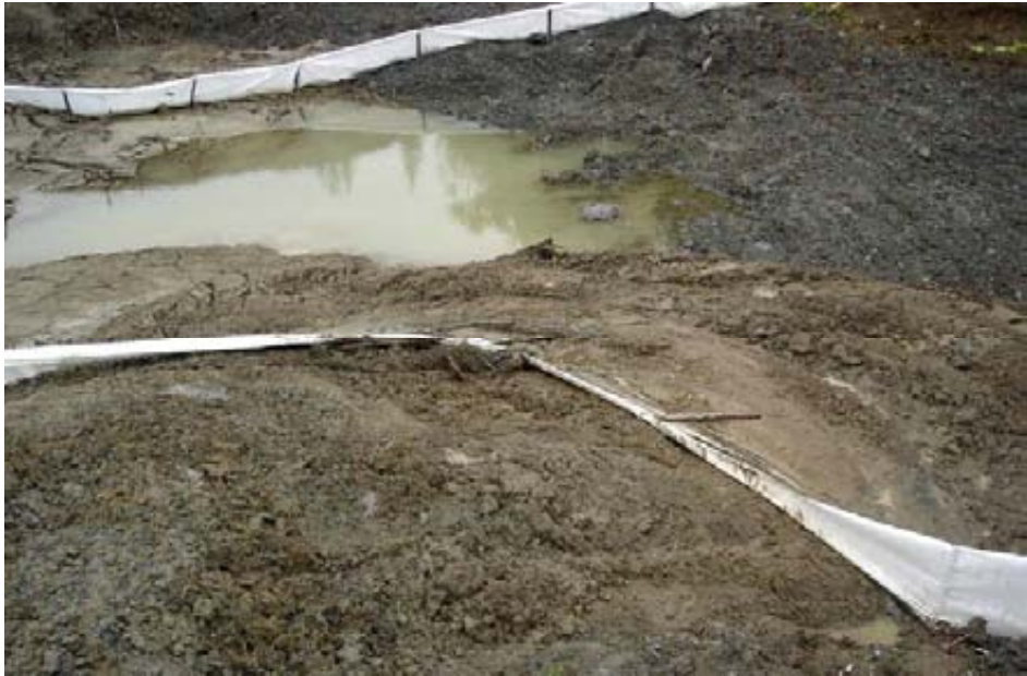
KP 461,0. The landslide on the right bank of Krasnaya River (the same place as on the previous slide). The photos above and below show that silt protection screens made of geotechnical fabric are mounted directly on the moving “bodies” of the landslides moving to the waterways. Photo above to the right - there is slush moving instead of the water. July 2, 2007.
