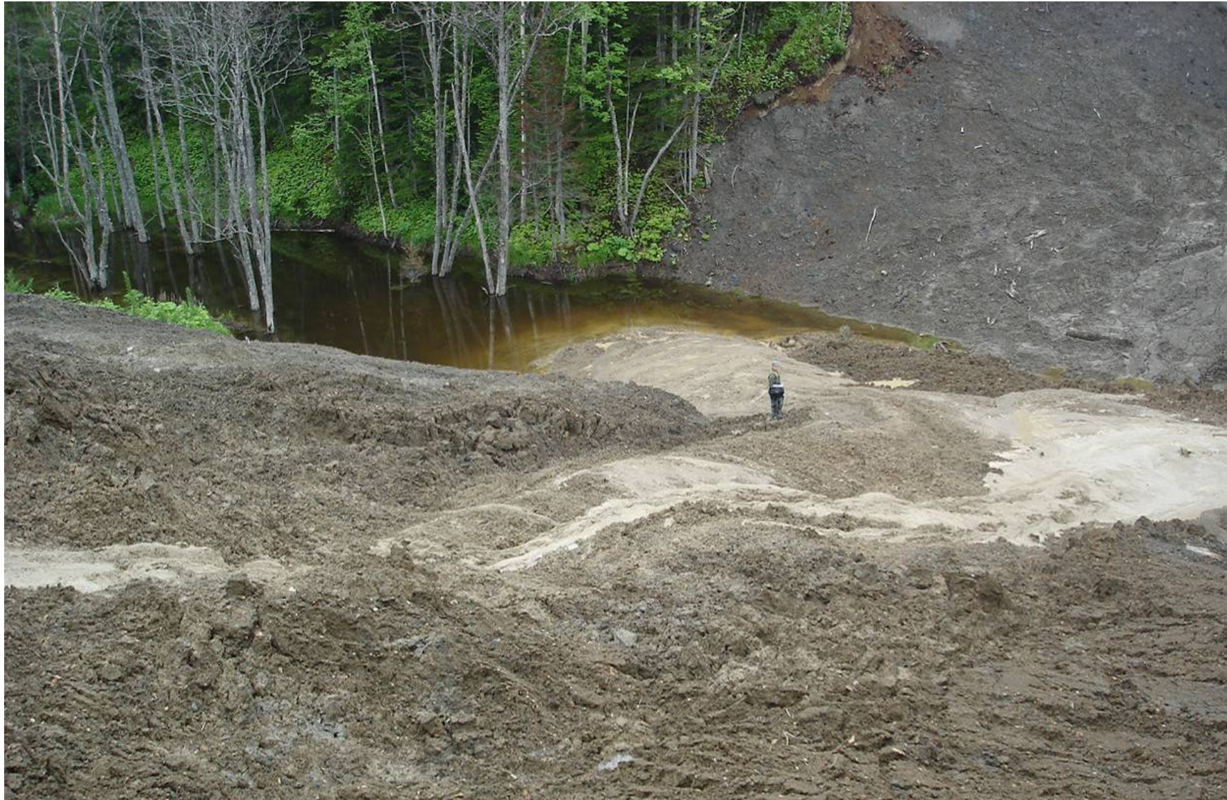
KP 462,6. A landslide on the right bank of the left tributary of the Baklanovka River, Dolinsk District. (the same place as on the previous slide). The landslide completely blocked the stream's bed, blocking water flow. An artificial pond has been created. Hydrological regime of the waterways was violated. Obviously, during water flooding considerable volumes of soil will be washed down the spawning Baklanovka River. July 2, 2007.
