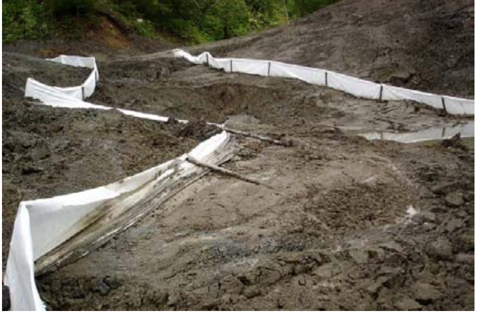
KP 461,0. The landslide on the right bank of Krasnaya River (the same place as on the previous slide). The photos above and below show that silt protection screens made of geotechnical fabric are mounted directly on the moving “bodies” of the landslides moving to the waterways. Photo above to the right - there is slush moving instead of the water. July 2, 2007.
