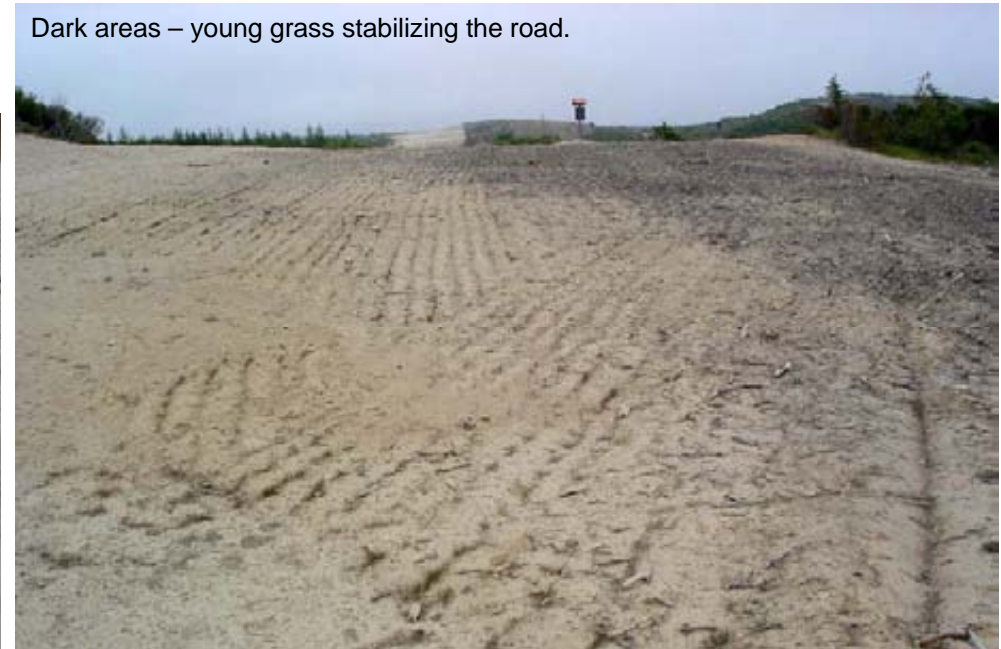
The grass under the cloth is coming remarkably well. In few years it will play stabilizing role instead of decomposed cloth.
