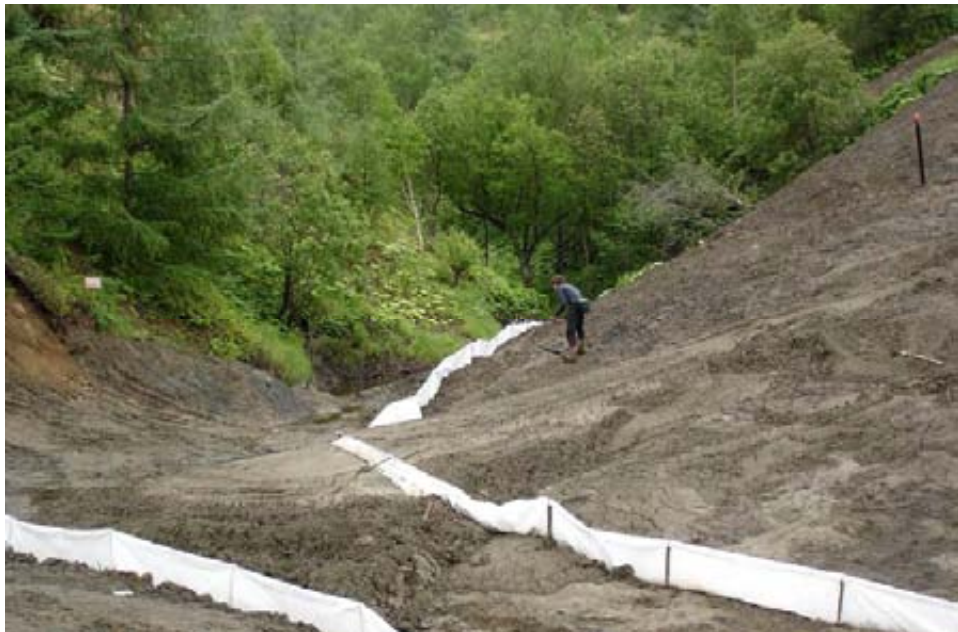
KP 461,0. The landslide on the right bank of Krasnaya River (the same place as on the previous slide). The photos above and below show that silt protection screens made of geotechnical fabric are mounted directly on the moving “bodies” of the landslides moving to the waterways. Photo above to the right - there is slush moving instead of the water. July 2, 2007.
