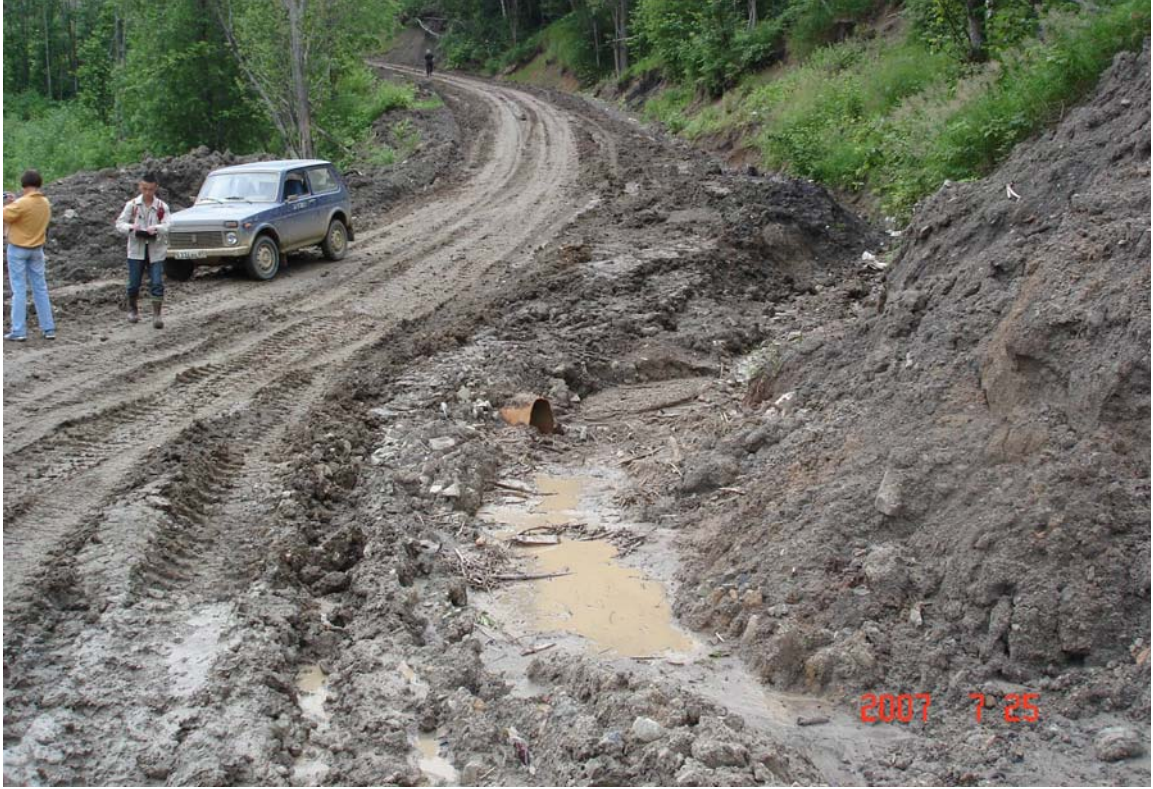
Right shore of the Krinka River. Roadside ditches along the access road, which drain into the river.
