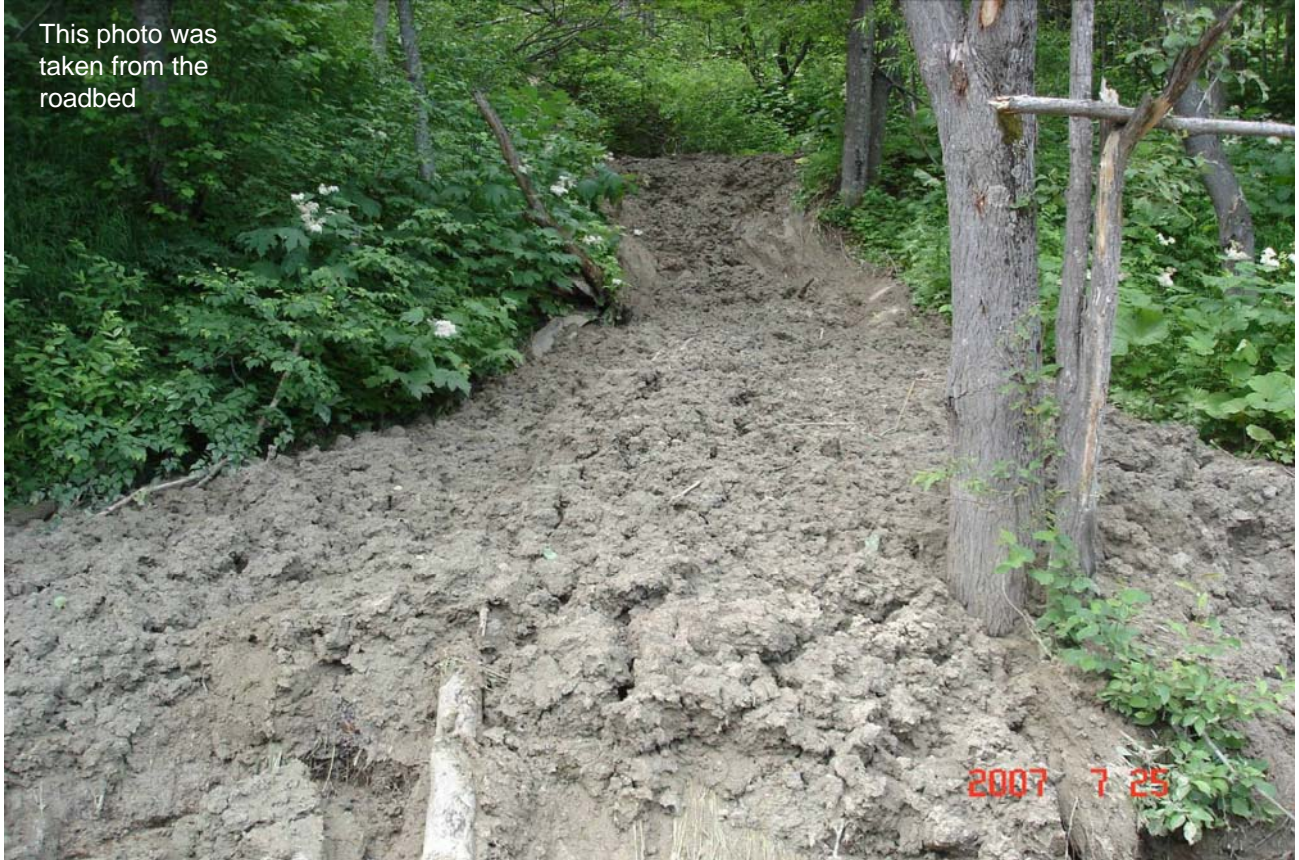
July 25, 2007. A mudflow about 100 meters in length, flowing down from the pipeline route along a forested slope of a mountain down to the access route, in a section that is adjacent to the right shore of the Krinka River.
