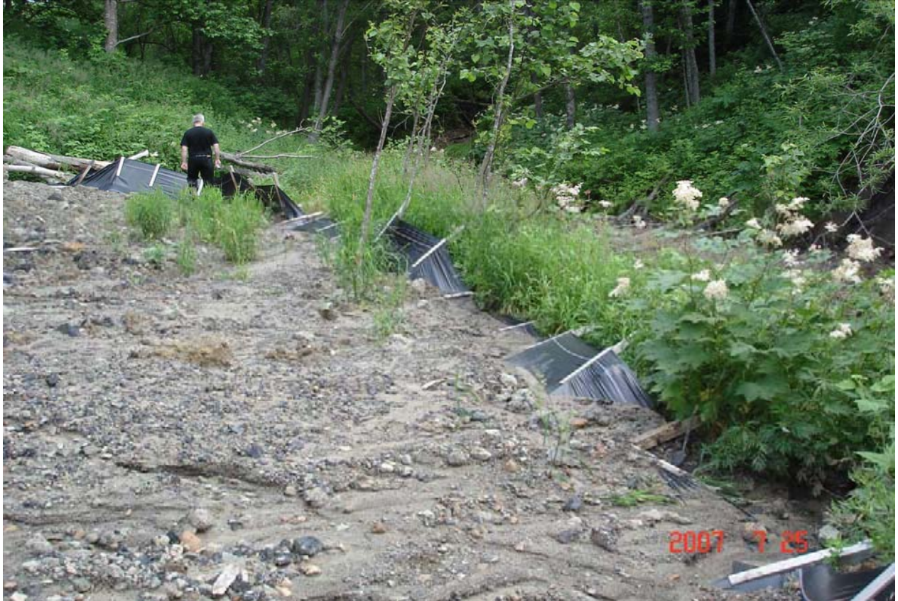
Un-numbered stream, KP 349.18. Upstream (upper photo) and downstream (lower photo) from the temporary bridge. Anti-sludge screens are destroyed and have not been repaired.
