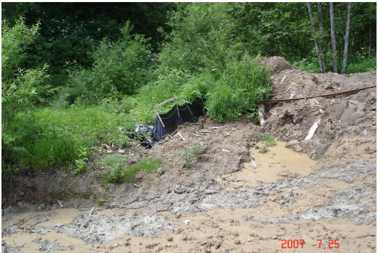
Un-numbered stream, KP 349.18. Upstream (upper photo) and downstream (lower photo) from the temporary bridge. Anti-sludge screens are destroyed and have not been repaired.
