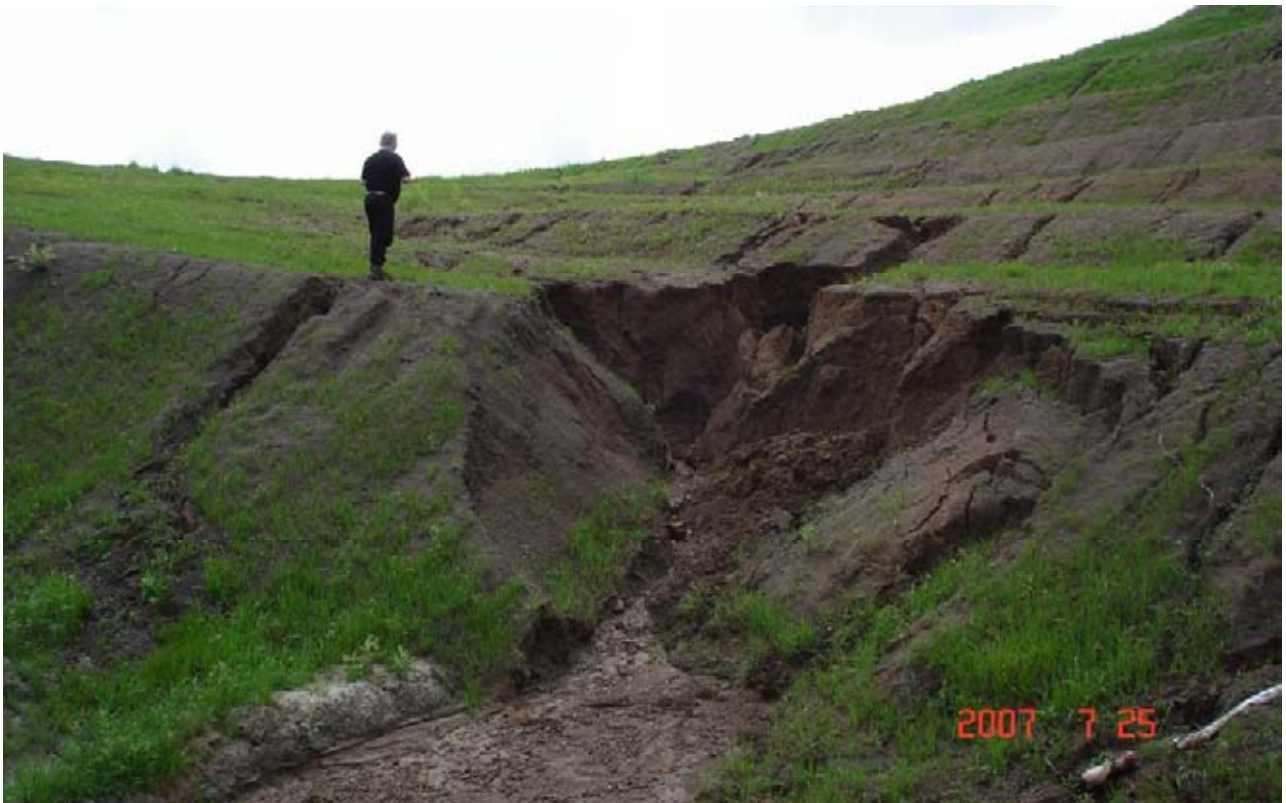
July 25, 2007. A section of the Krinka River watershed and its right tributary (Left Krinka), downstream from the pipeline route. A pile of waste construction soil that was extracted from the pipeline route, beyond the right-of-way. Despite the terracing of the slope and planting of grass, erosion is beginning on the pile.
