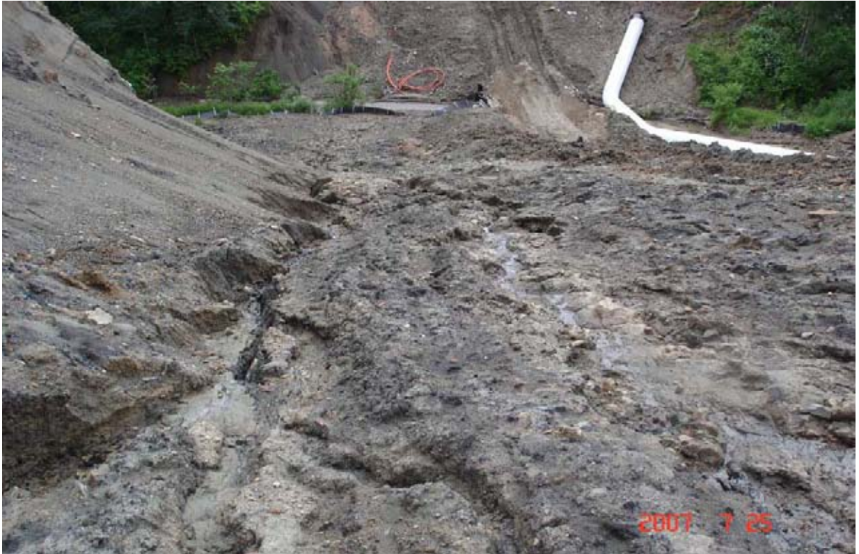
July 25, 2007. Un-numbered stream, right tributary of the Krinka River of the 1 st order, a reservoir of the highest (special) category in terms of fisheries value. The area for salmon spawning in range of the river-crossing until the start of construction consisted of 44 m 2 . The location of the river-crossing is at KP 349.18. In the background on the right one can see a length of gas pipeline that is ready to be buried. In the background on the left is erosion wash-out
