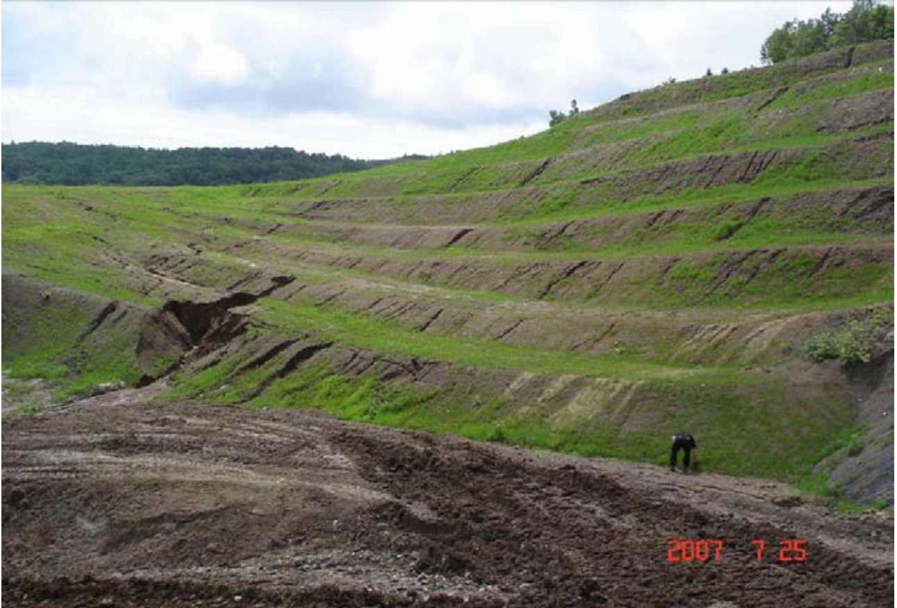
July 25, 2007. A section of the Krinka River watershed and its right tributary (Left Krinka), downstream from the pipeline route. A pile of waste construction soil that was extracted from the pipeline route, beyond the right-of-way. Despite the terracing of the slope and planting of grass, erosion is beginning on the pile.
