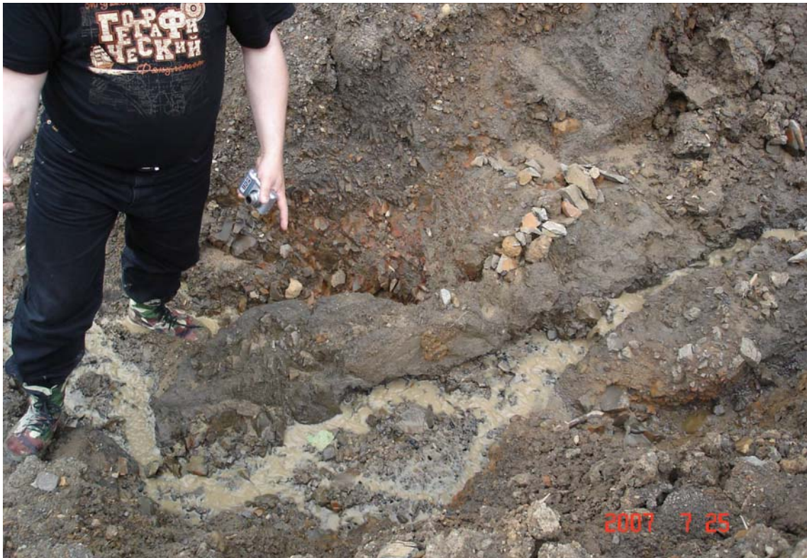
Left shore of the Krinka River, river valley slope. Active erosion processes on the pipeline route. Excavation in this section has been going on since 2005, although anti- erosion measures on the slope have been absent during this entire time.
