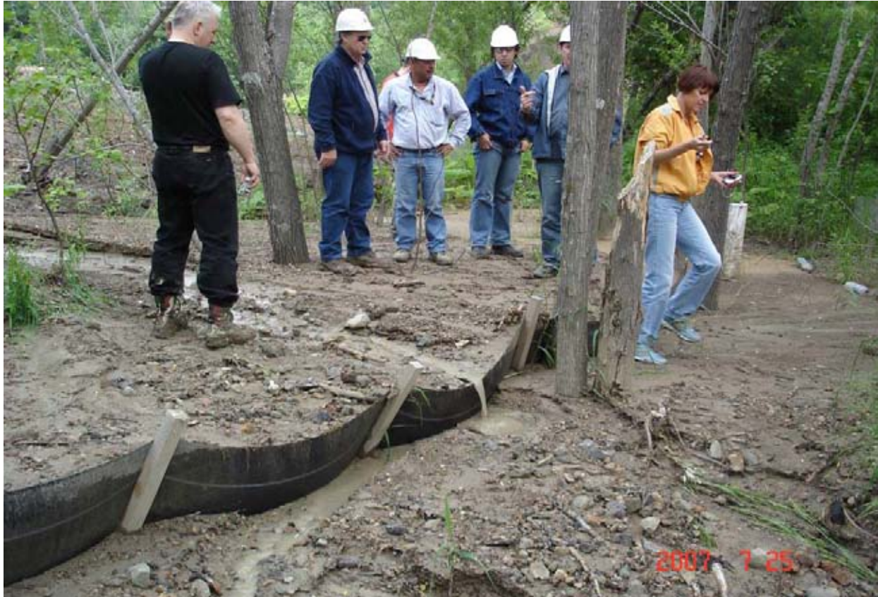
Right shore of the Krinka River, below the pipeline river-crossing. A large amount of sludge sediments on The protected shoreline zone, which is overflowing the projective screens. Unauthorized occupation of the forest in a water-protection zone, beyond the right-of-way.
