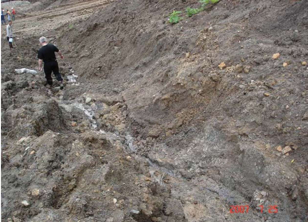
Left shore of the Krinka River, river valley slope. Active erosion processes on the pipeline route. Excavation in this section has been going on since 2005, although anti- erosion measures on the slope have been absent during this entire time.
