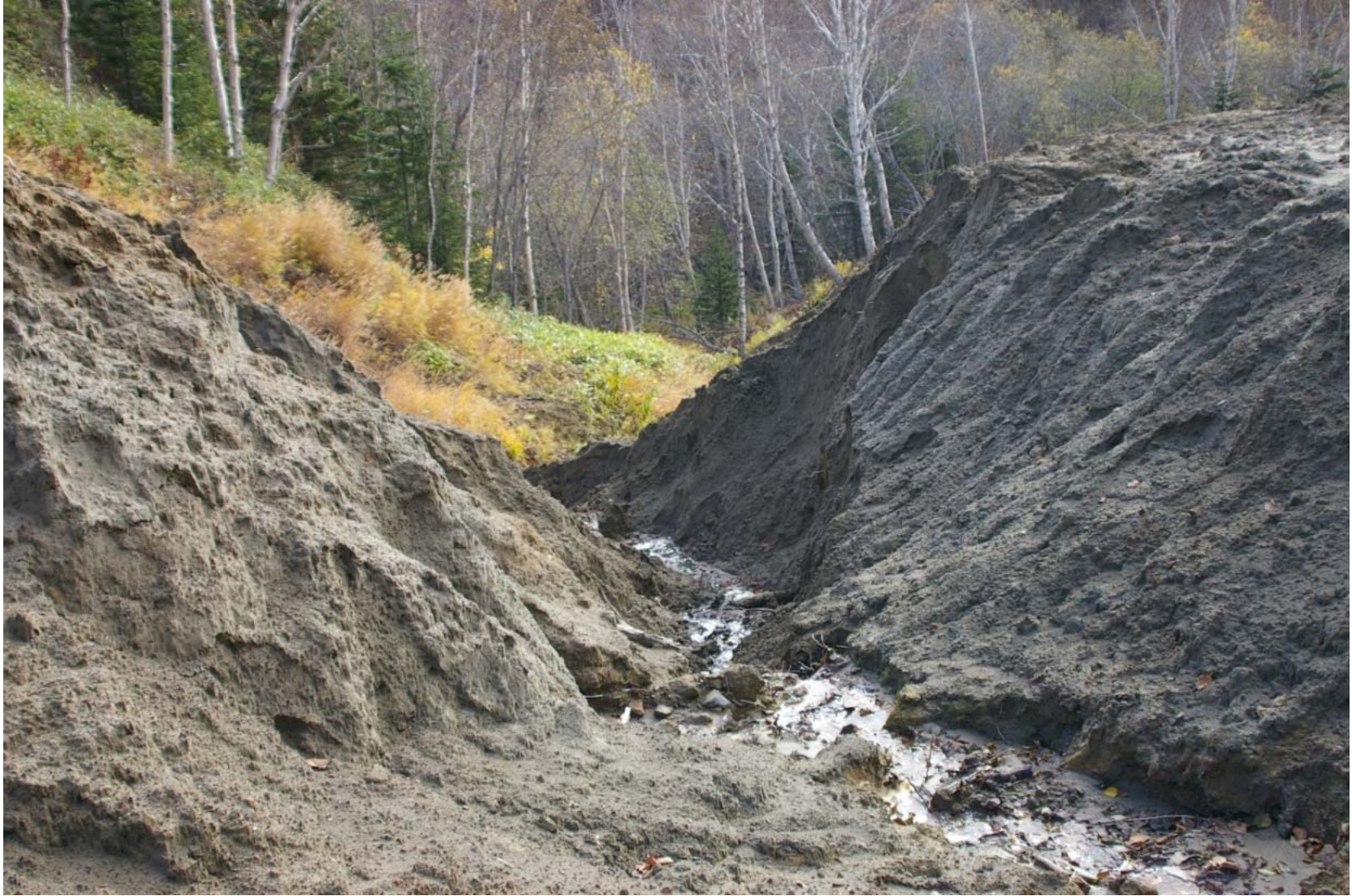
October 23, 2007: KP 492.4. An earth mound which was washed out by the stream.
