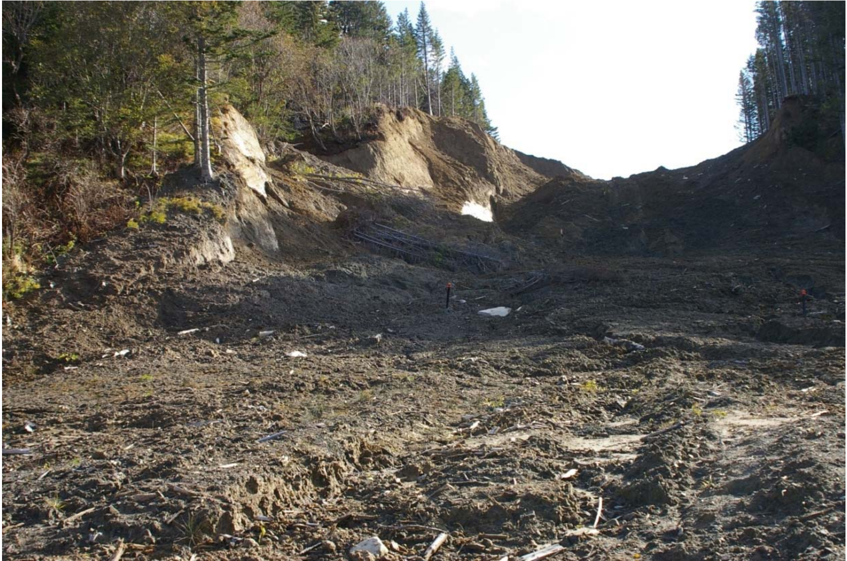
October 23, 2007: KP 482.5. The right bank of the Primorskaya River. A significant land slide.
