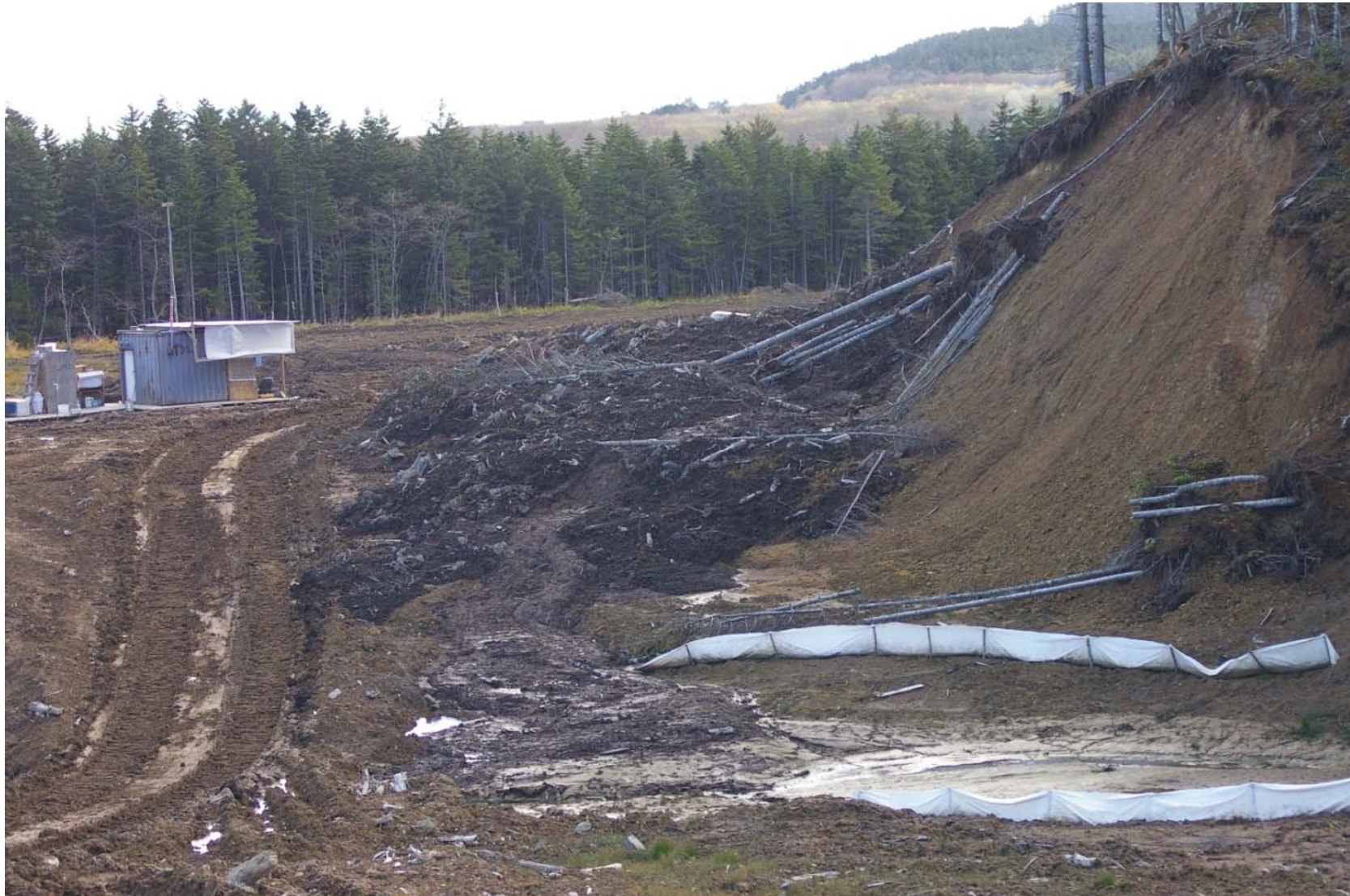
October 23, 2007: KP 483.7. Trees and soil have covered the RoW next to a stream to the north of Firsovo Village.
