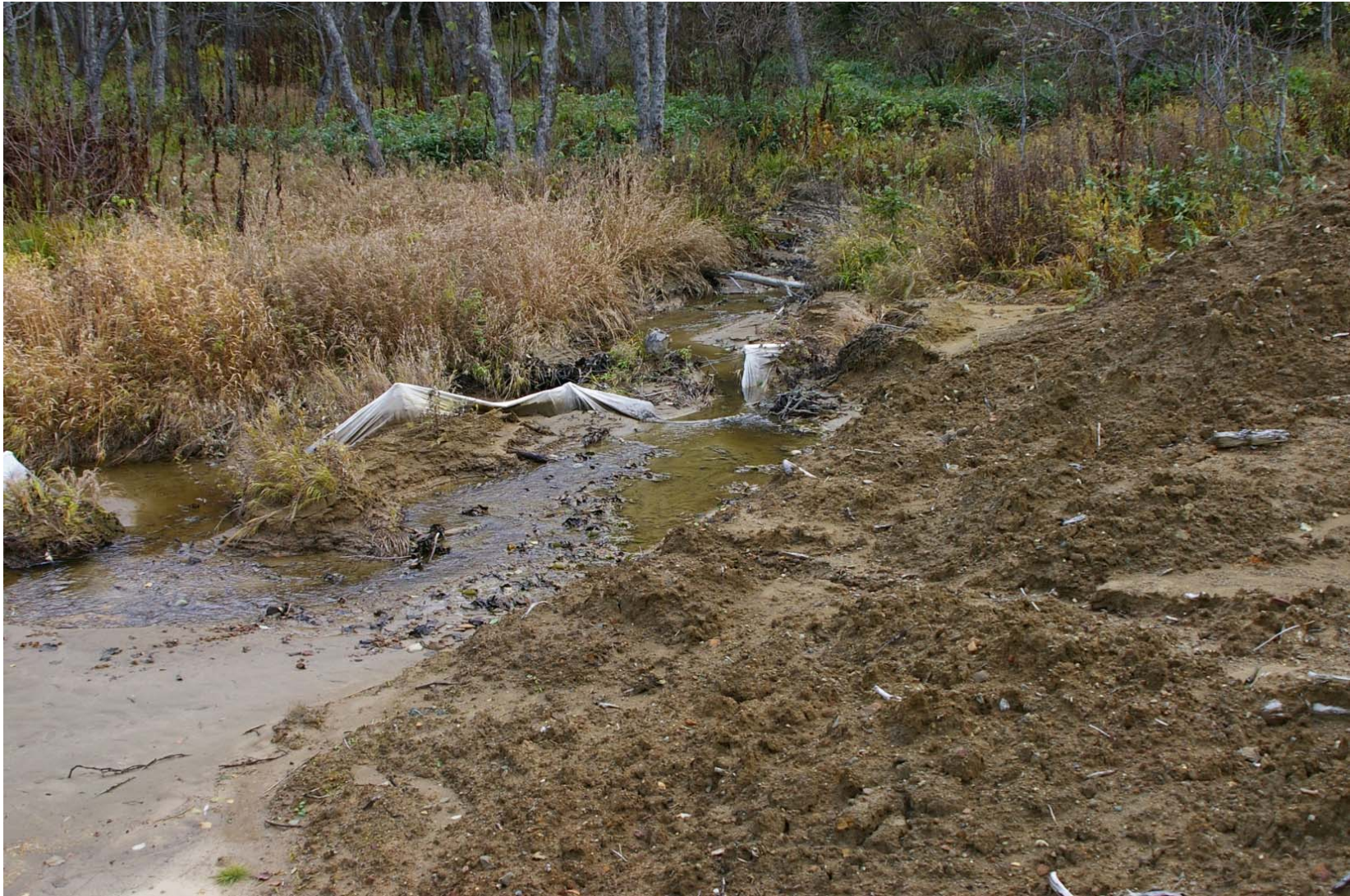
October 23, 2007: KP 493.7. The stream to the south of the Listvennitsa River. Mud enters the stream and anti-erosion silt fences have been abandoned since autumn 2006.
