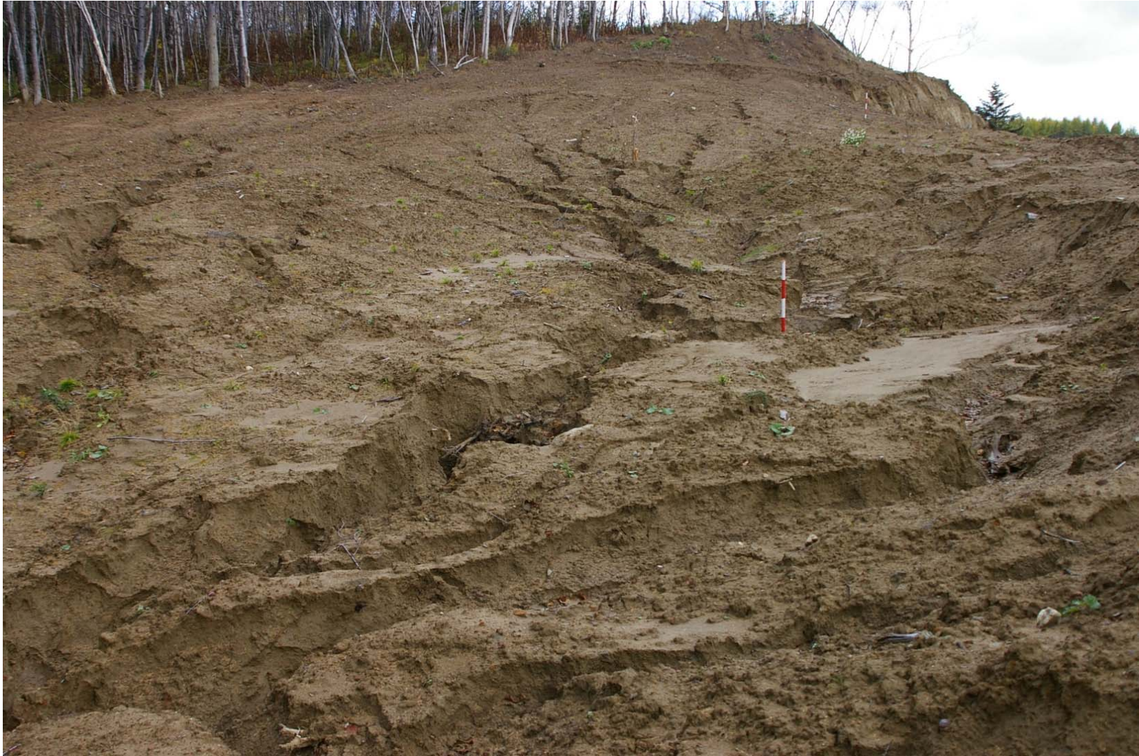
October 23, 2007: KP 493.2. 300 meters to the south of the Listvennitsa River. Erosion ditches on the pipeline RoW.
