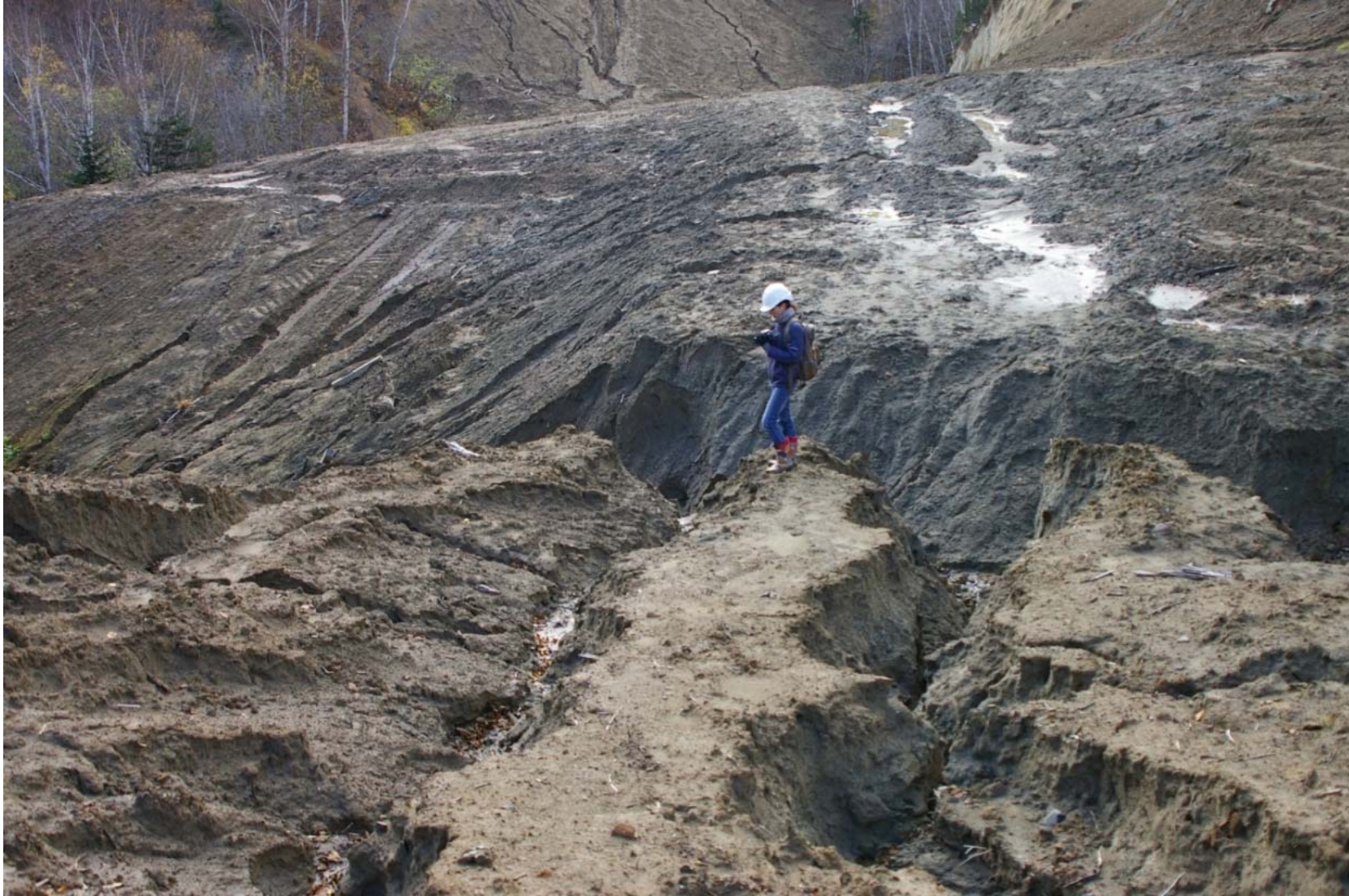
October 23, 2007: KP 492.4. Left tributary of the previous stream (to the north of the Listvennitsa River). This small stream was also blocked by an earth mound in the winter and has since passed through the mound, causing serious erosion processes.
