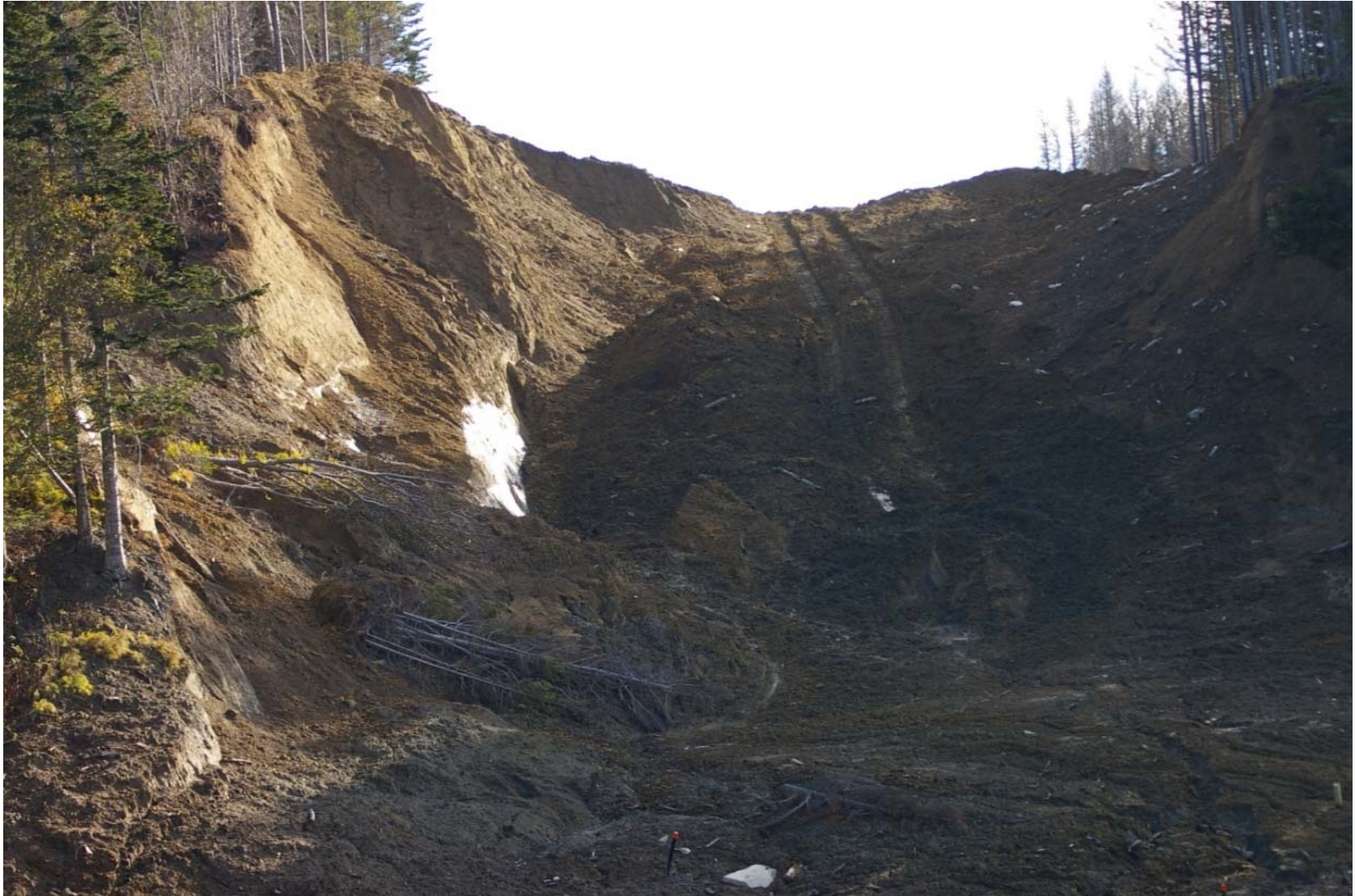
October 23, 2007: KP 482.5. The right bank of the Primorskaya River. A significant land slide.
