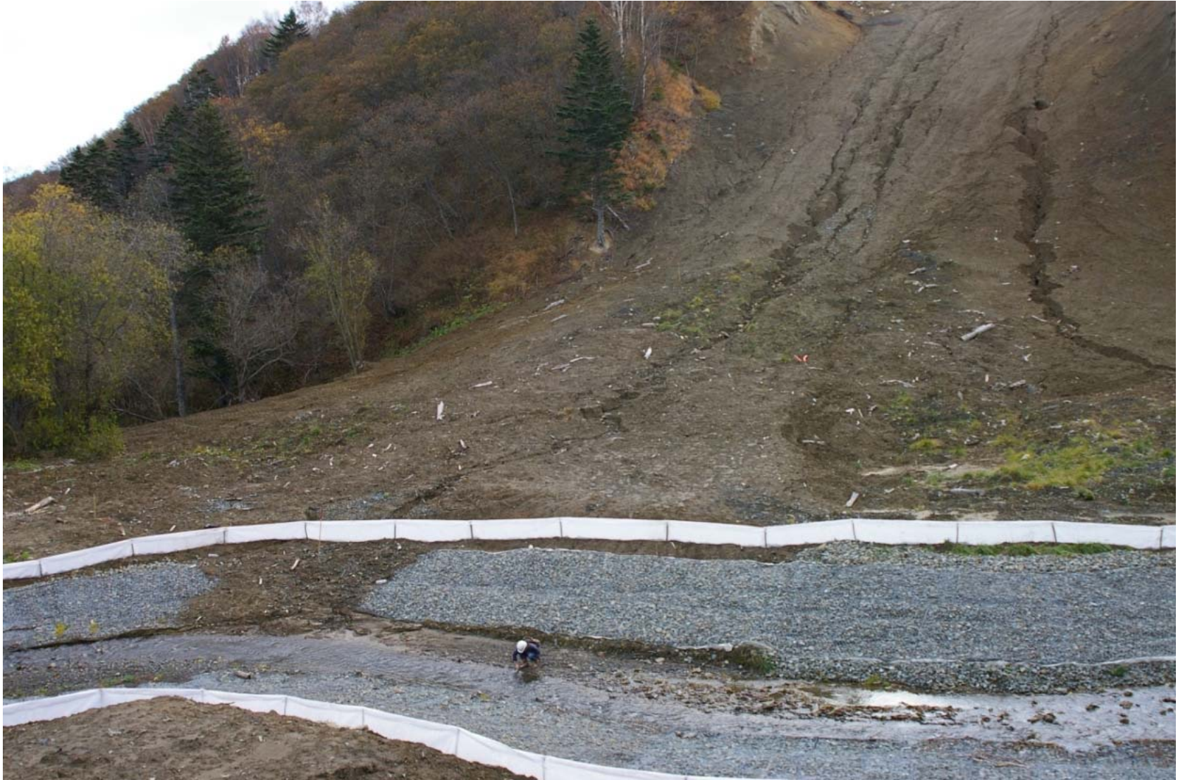
October 23, 2007: KP 489.5. The right bank of the Rybnaya River where mudflows crossed Reno mats into the river.
