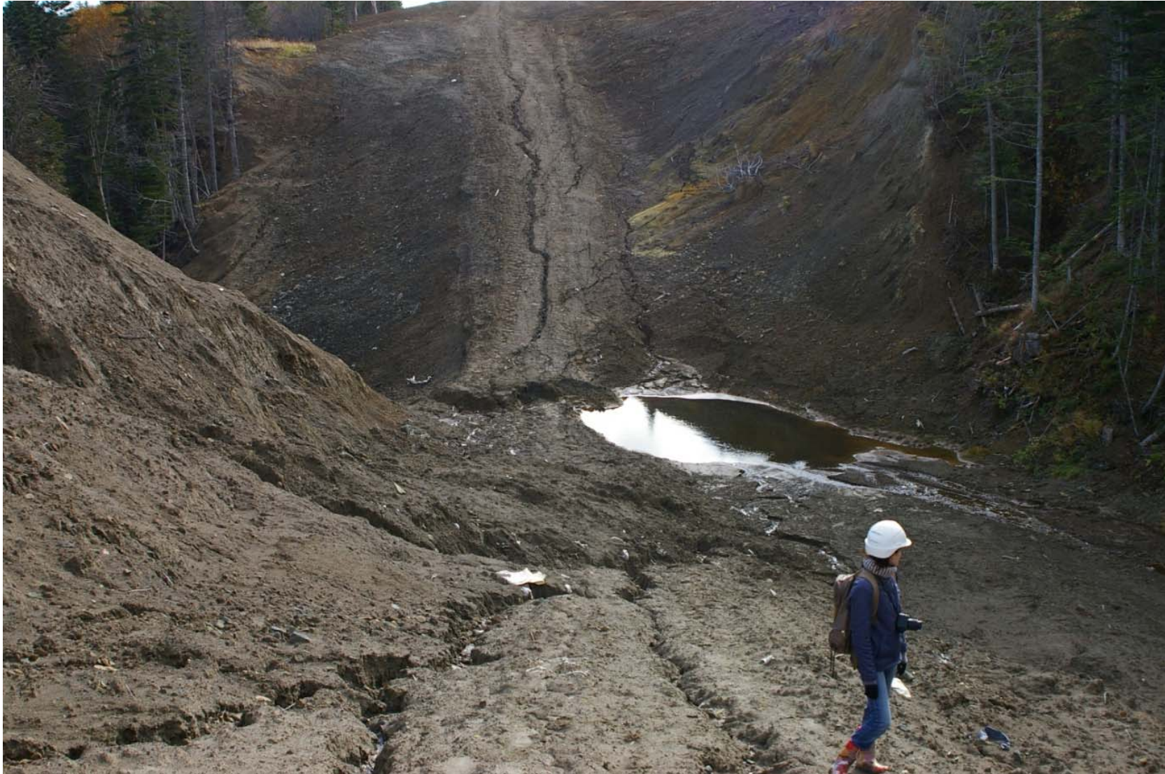
October 23, 2007: KP 490.6. Erosion runoff enters the stream to the north of the Krutoyarka River.
