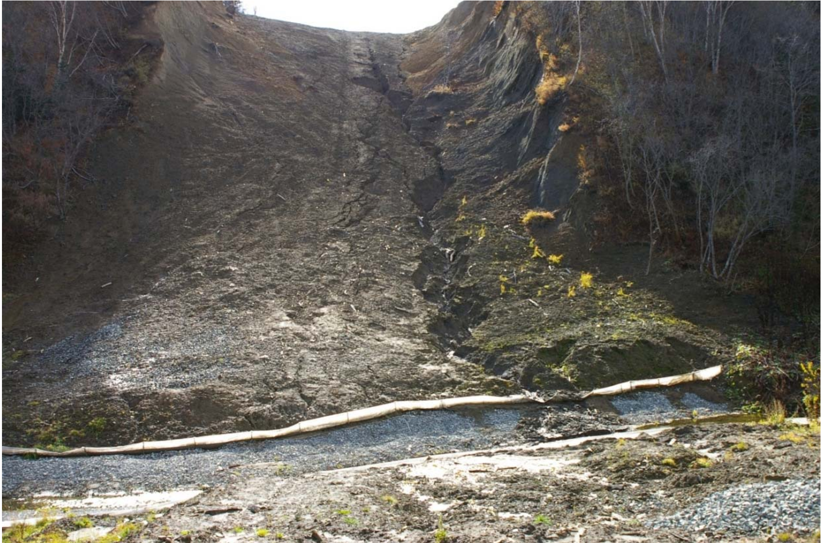
October 23, 2007: KP 491.4. Right bank of the Krutoyarka River.
