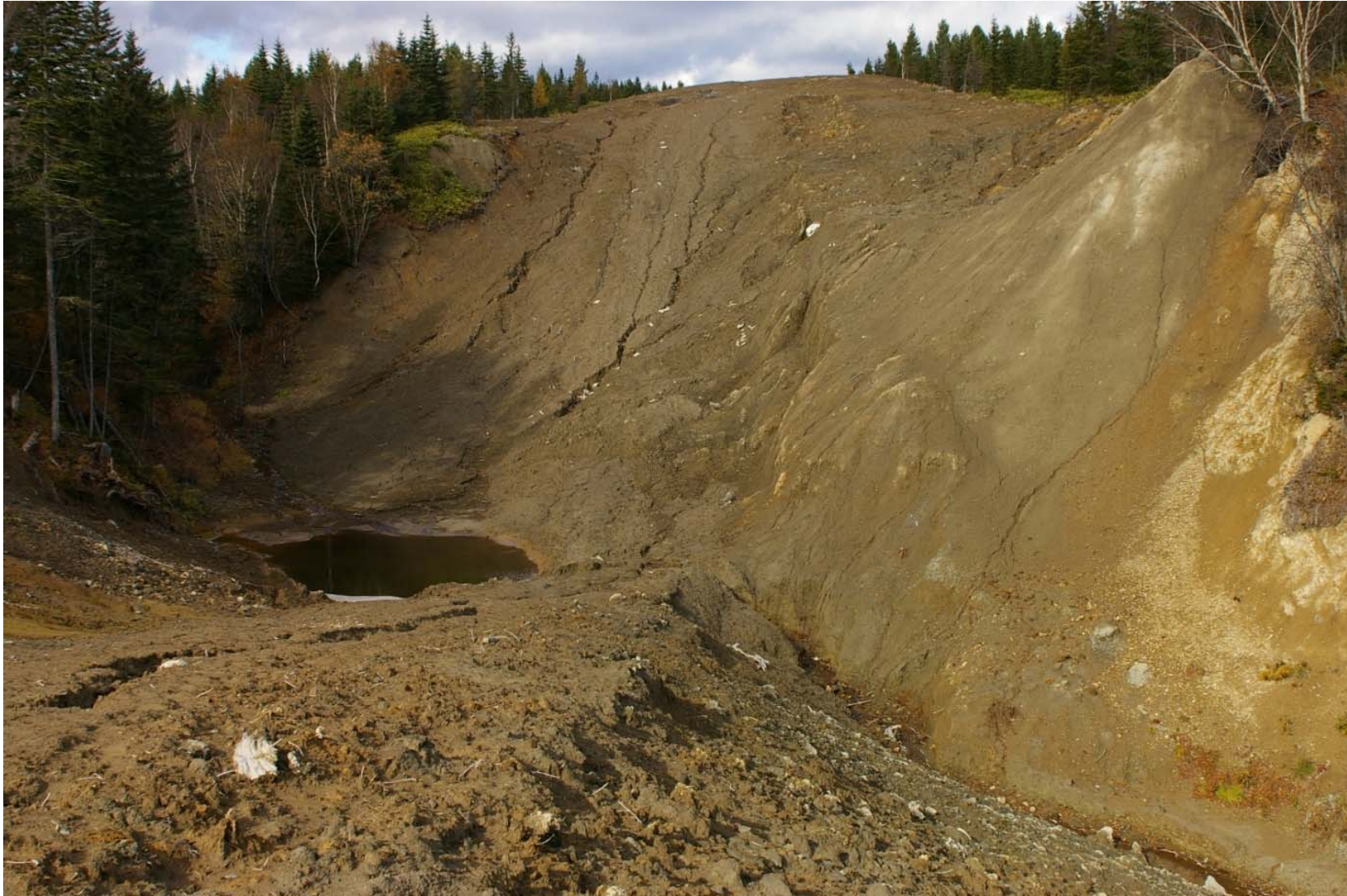
October 23, 2007: KP 490.6. Stream to the north of the Krutoyarka River. The pond formed as a result of the stream flow being blocked by an earth mound.
