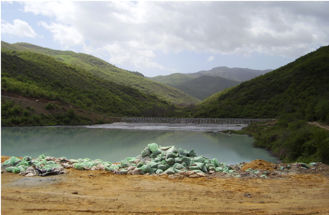
4) The up-stream part of the Geganush TMF, separated by earth embankment from the dry part
