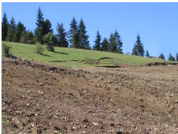
Landslide area in pipeline corridor
