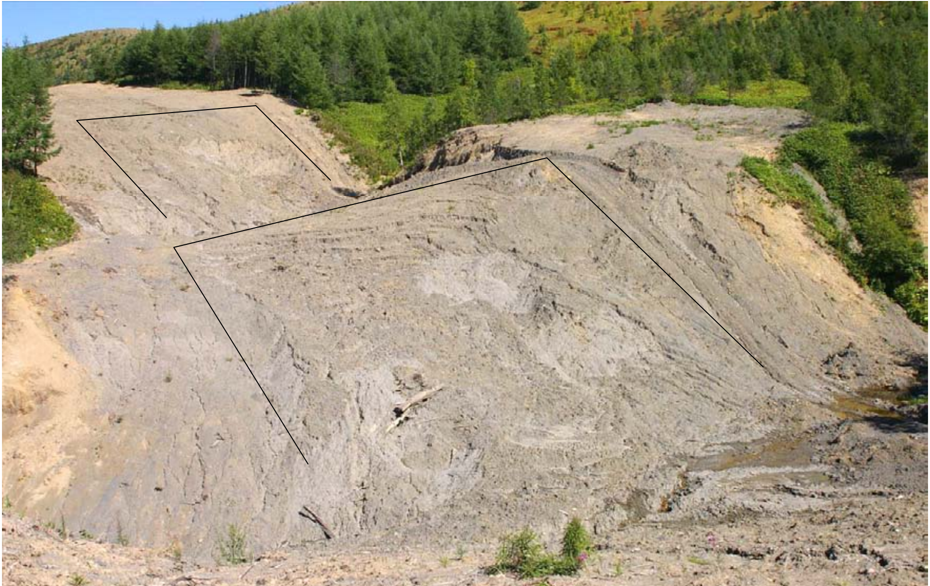
PK 461.6. The right tributary of the Krasnaya River, the right bank of the stream. Dolinsk District (the very site as the one on the preceding slide). Again, no protective measures at all. The landslide areas are marked with black lines. It is well seen that the situation is typical and is reoccurring. The soil sliding down into the stream is being continuously eroded; many tons of the muddy sediment have been polluting the spawning areas lying downstream. August 31, 2007.
