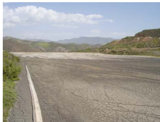
Dry tailings at the Geganush tailings facilities
