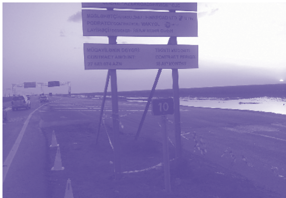
▲ A section of the Baku to western Shamakhi District road
