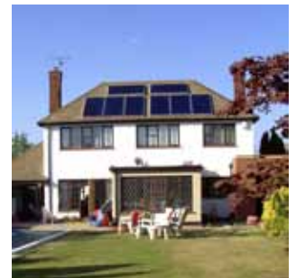
Photo: Watt S.A.
