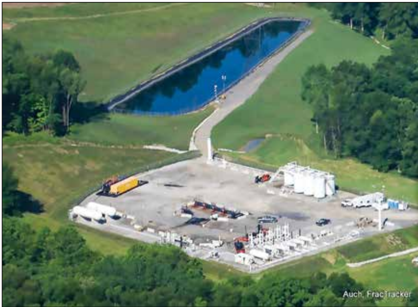
Utica field, Ohio, USA. Drilling platform with six wells, a compressor station and fracking fluid storage pit.
