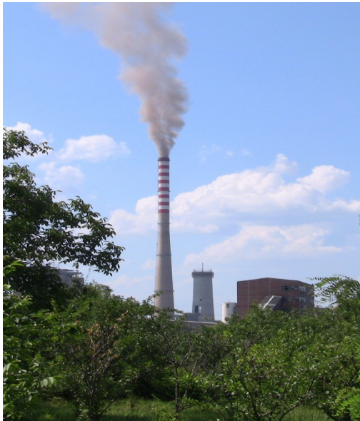
Illustration 2: Chimney photographed on July 16 2015 (construction to the right of main chimney)
