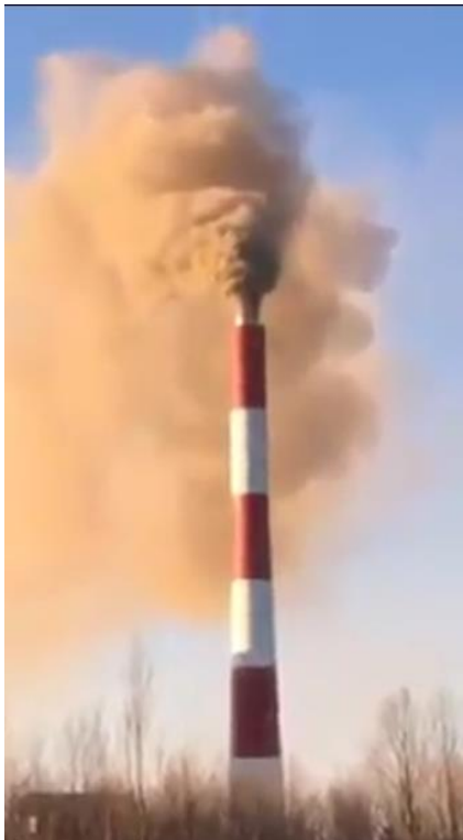
Stanari power plant, January 2018, photo capture: https://www.facebook.com/221561244645441/videos/1209652729169616/
