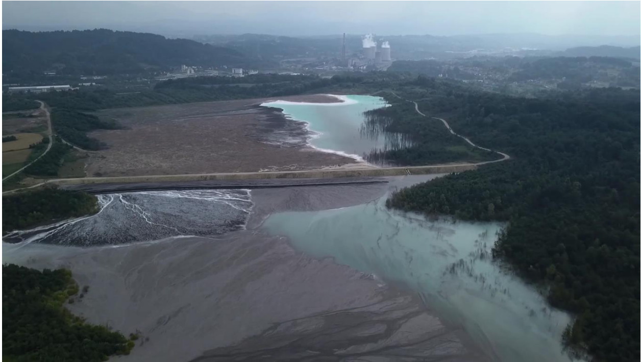
Tuzla ash disposal site and power plant in the background, photo capture: https://www.facebook.com/CentarZaZivotnuSredinu/videos/551026885345677/
