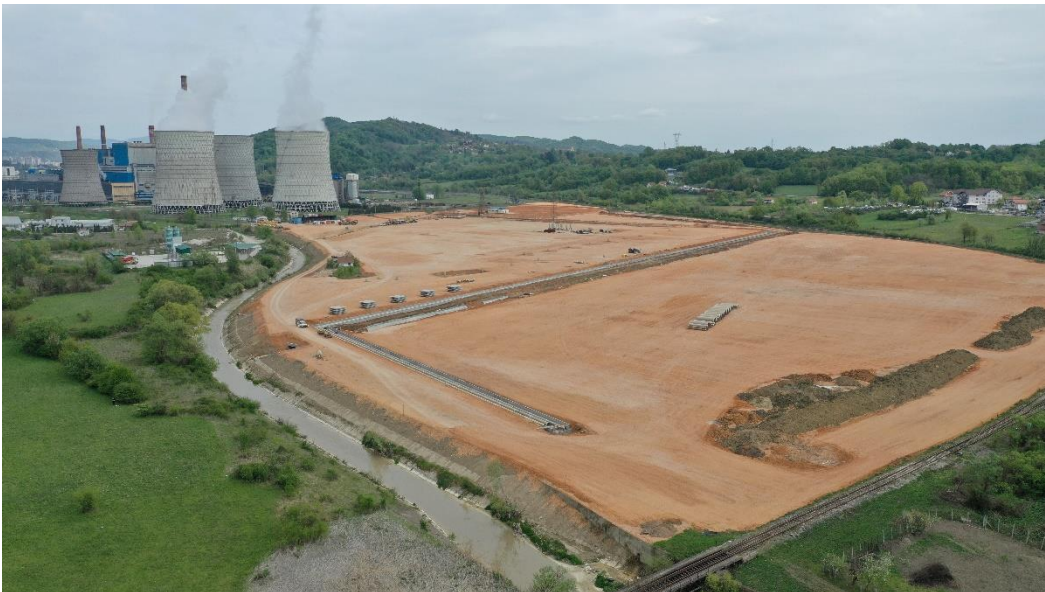
Preparation works for Tuzla 7. Photo: Denis Žiško
