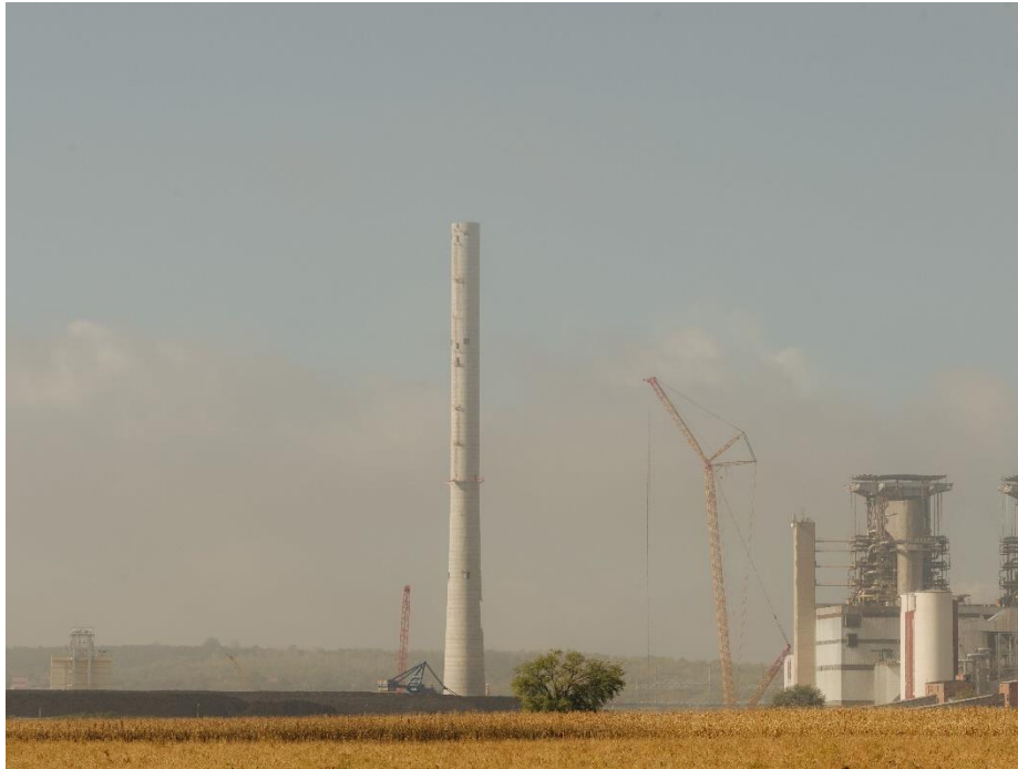
Kostolac B3 under construction. Photo: Dan Wilton / ClientEarth
