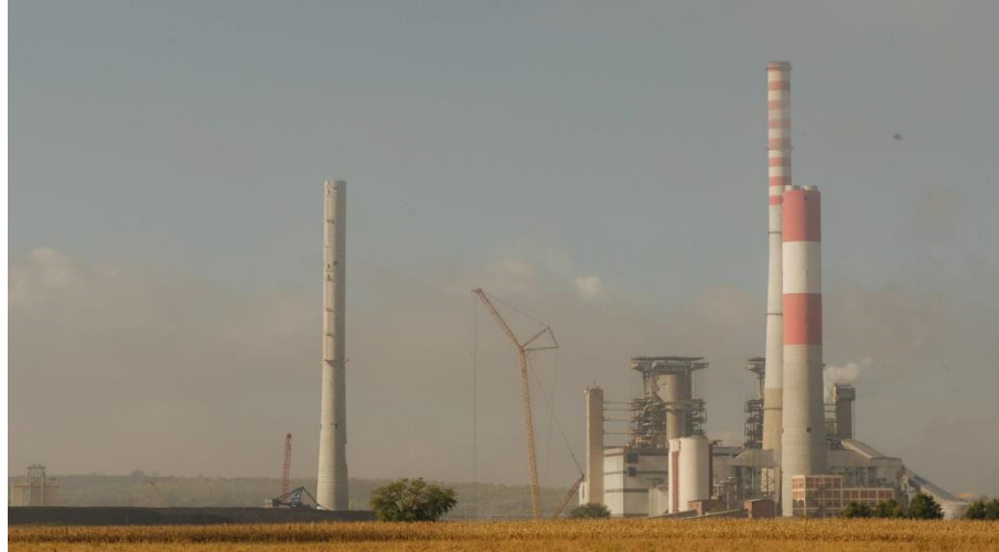
The Kostolac B3 chimney under construction and the disfunctional de-SOx chimney Credit: Dan Wilton / ClientEarth
