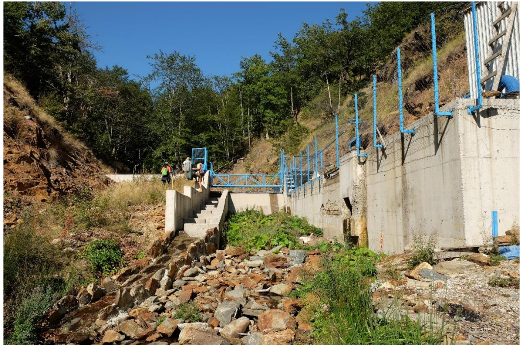
Almost dry fish pass and riverbed below Brajcino 1 intake, North Macedonia Photo: Igor Vejnović
