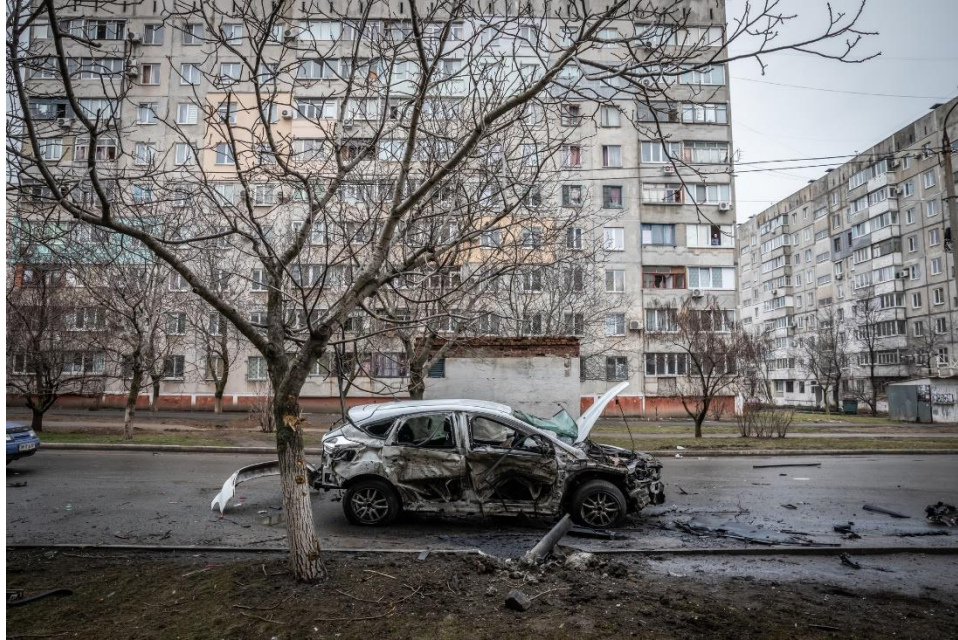
Soviet-style residential blocks in Mariupol, now destroyed. Photo by darvik.photography@gmail.com via depositphotos.
