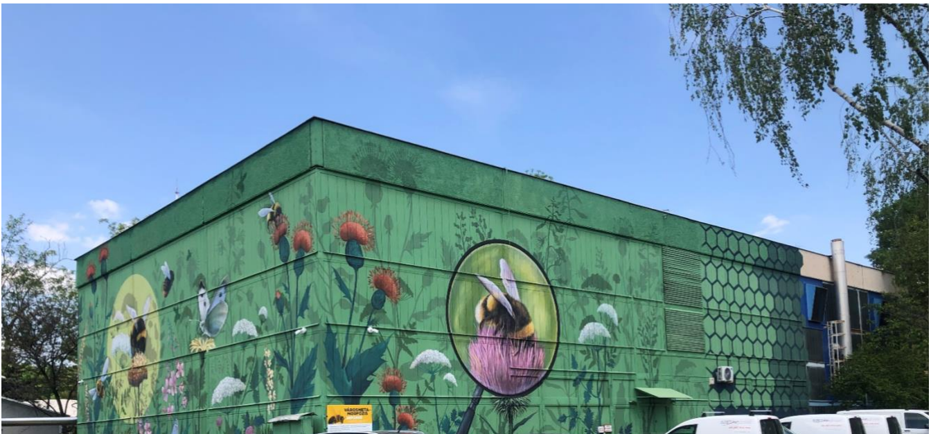
Geothermal heating plant in Szeged, Hungary
