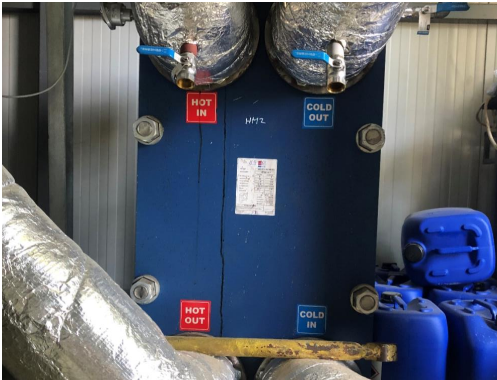
Geothermal water pipes in Szetav, Hungary
