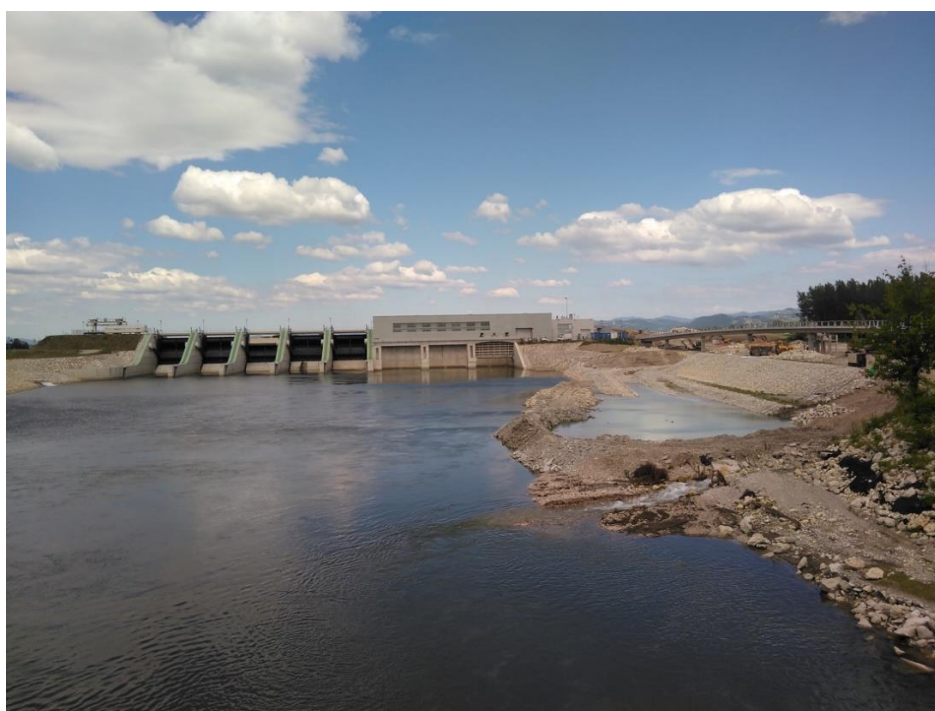
The Brežice hydropower plant on the river Sava in Slovenia. Photo taken by the author
