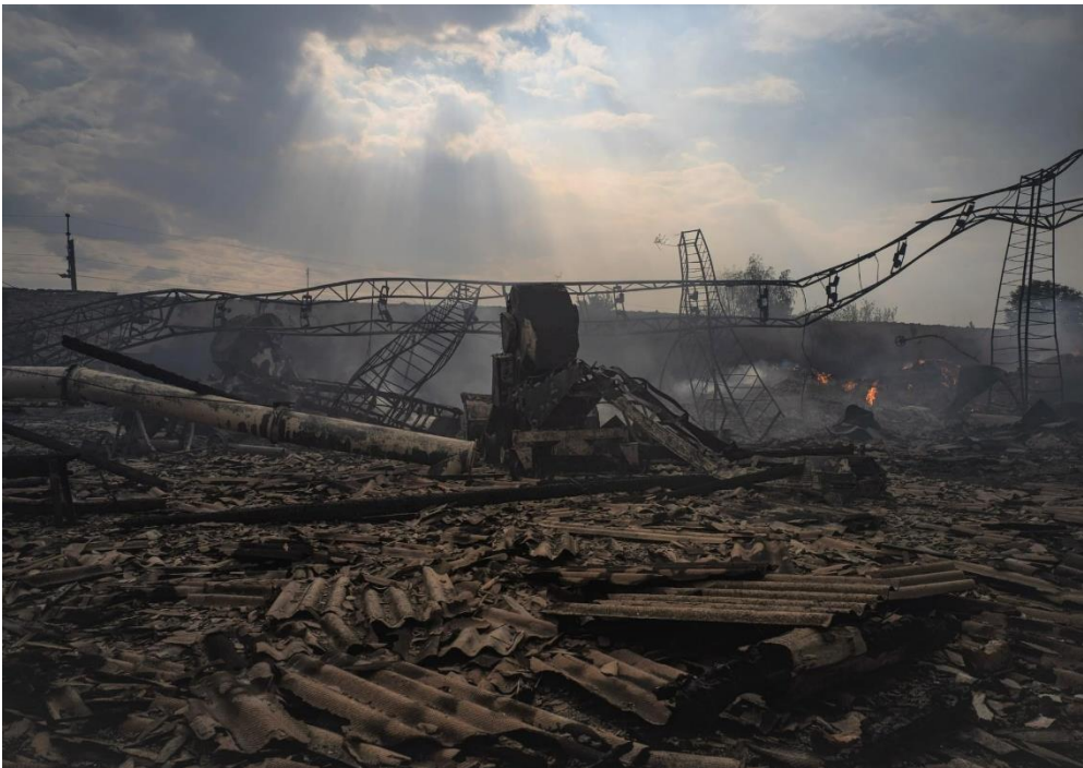
Destroyed transmission line, Siversk, May 2022. Photo by Kurekaoru
