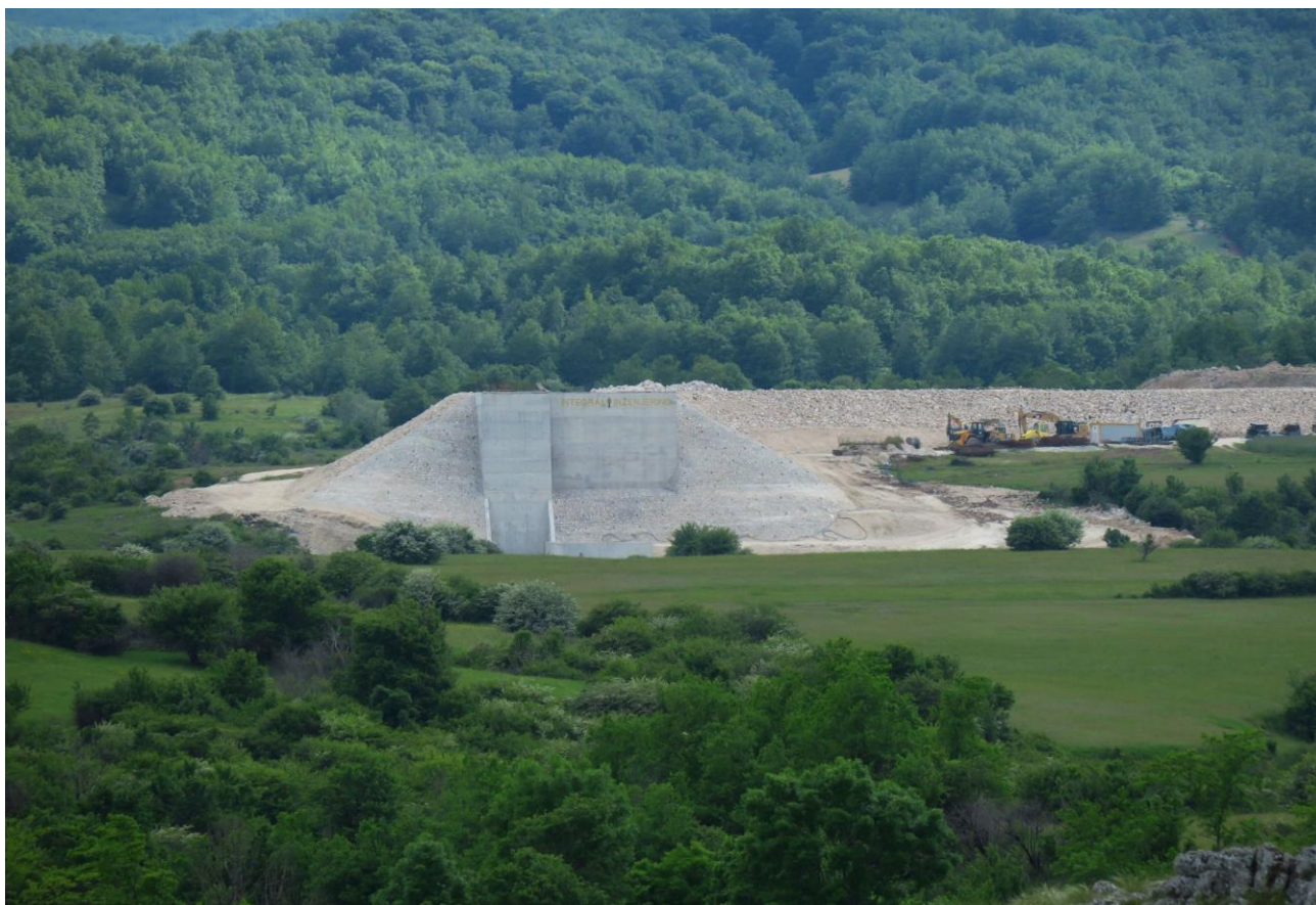
The entrance to the tunnel at Nevesinjsko polje in the Zalomka river valley. Photo: CEE Bankwatch Network, June 2023.
