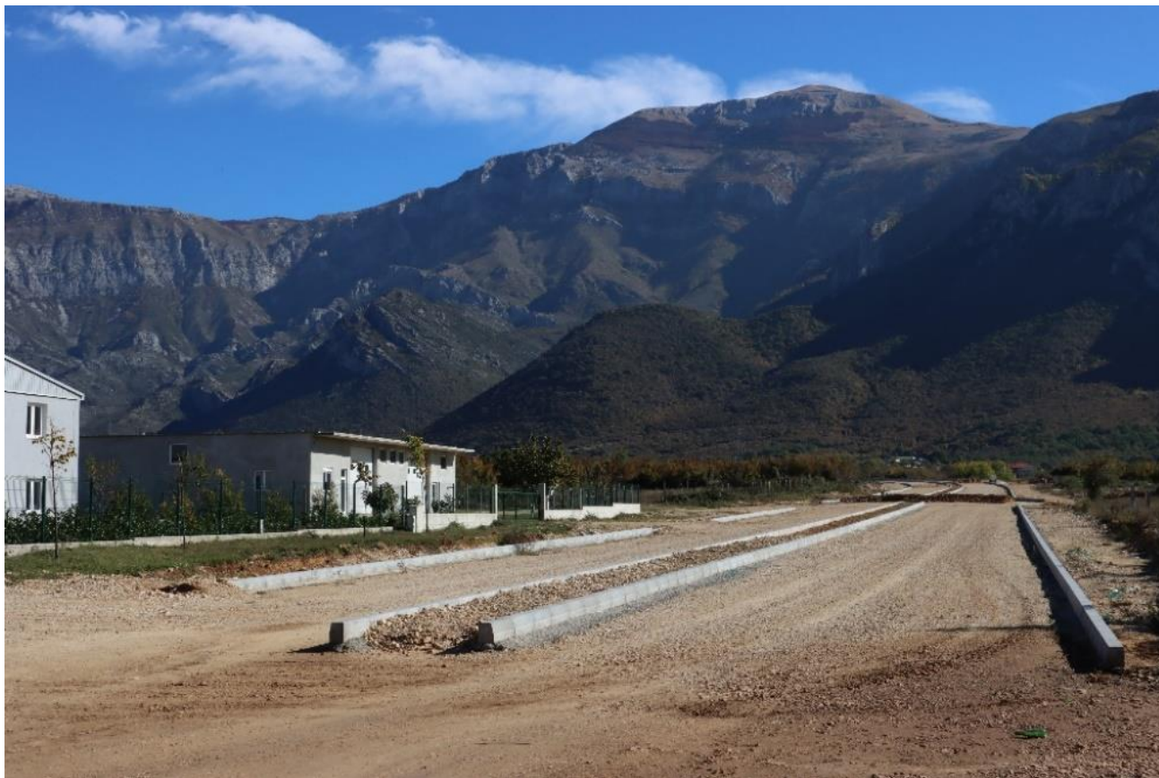
Construction of the Corridor Vc. Photo: CEE Bankwatch Network
