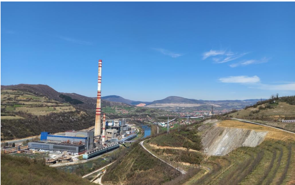
Kakanj power plant, Bosnia and Herzegovina, Photo: CZZS
