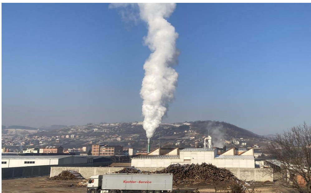
Biomass plant in Novi Pazar, Serbia (photo: Dragan Maksimovic).
