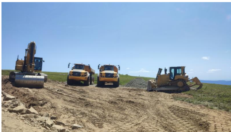
Construction activity underway on Mount Runa, 21 June 2025 (photo: CEE Bankwatch Network).
